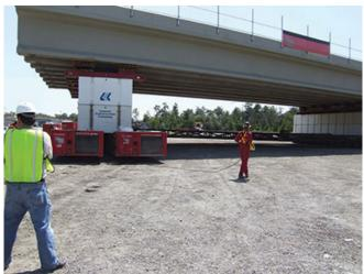
Example of Self-Propelled Modular Transporters (SPMT)
